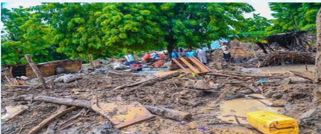
Figure 1.1 Flood damage in Yobe, Nigeria, July 2022. Photo Credits: State Emergency Management Agency in Yobe
